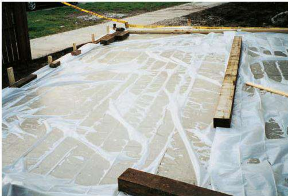
Figure 15-7. Polyethylene film is an effective moisture barrier for curing concrete and easily applied to complex as well as simple shapes. To minimize discoloration, the film should be kept as flat as possible on the concrete surface.
