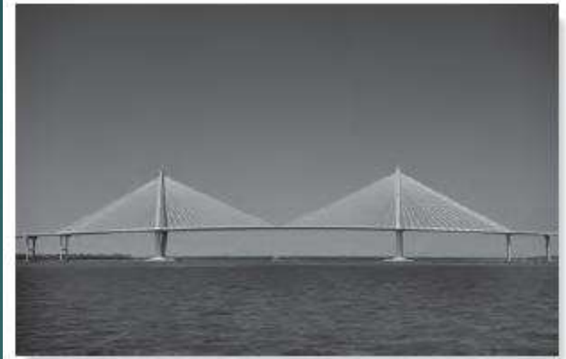
Cables support their loads in tension.
