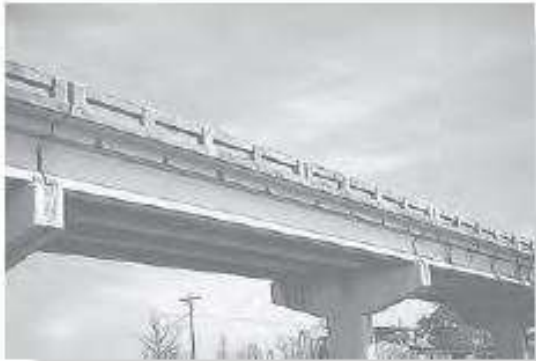
The prestressed concrete girders are simply supported and are used for this highway bridge.
