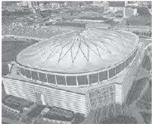
The roof of the “Georgia Dome” in Atlanta, Georgia can be considered as a thin membrane.
