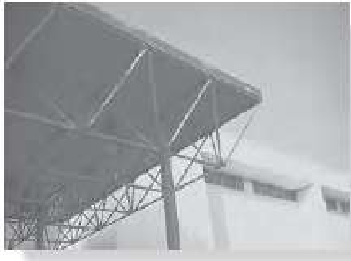
The roof of this pavilion is supported using a system of space trusses.
