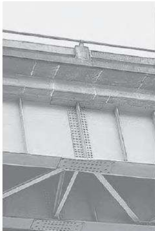
Shown are typical splice plate joints used to connect the steel girders of a highway bridge.
