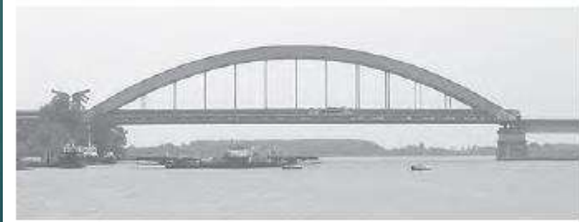
Arches support their loads in compression.
