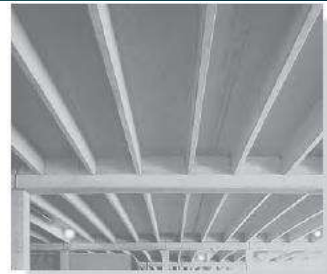
The structural framework of this building consists of concrete floor joists, which were formed on site using metal pans. These joists are simply supported on the girders, which in turn are simply supported on the columns.
